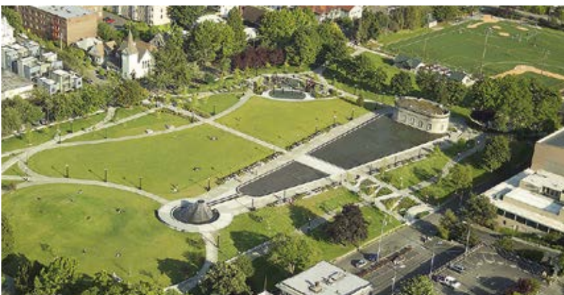
Lincoln Reservoir Cal Anderson Park SEATTLE, USA
